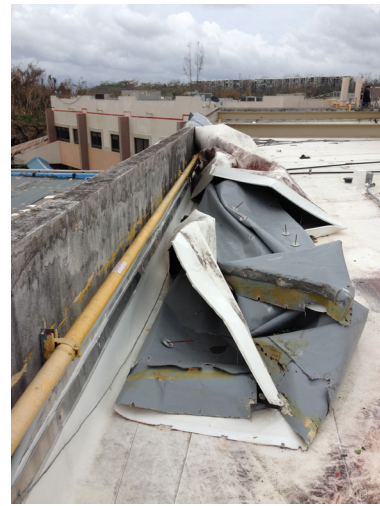
Maria uprooted trees and dumped a deluge of water on the roof of San Juan Capestrano Hospital's psychiatric center, which resembled a swimming pool during the storm. Shown here after being drained, the roof experienced significant damage, as did other structures on the hospital's campus.
